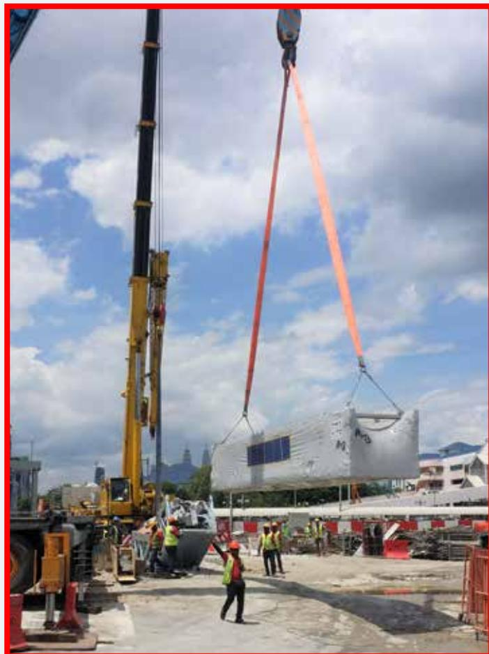
Due to constant changes in site, the lifting plan required several rounds of survey before the job could be performed. There were various obstructions so it took some planning to position the crane. Megalift also had to meet MMC-Gamuda's stringent requirements, particularly the crane utilisation part as they have their safety standards to be adhered.
