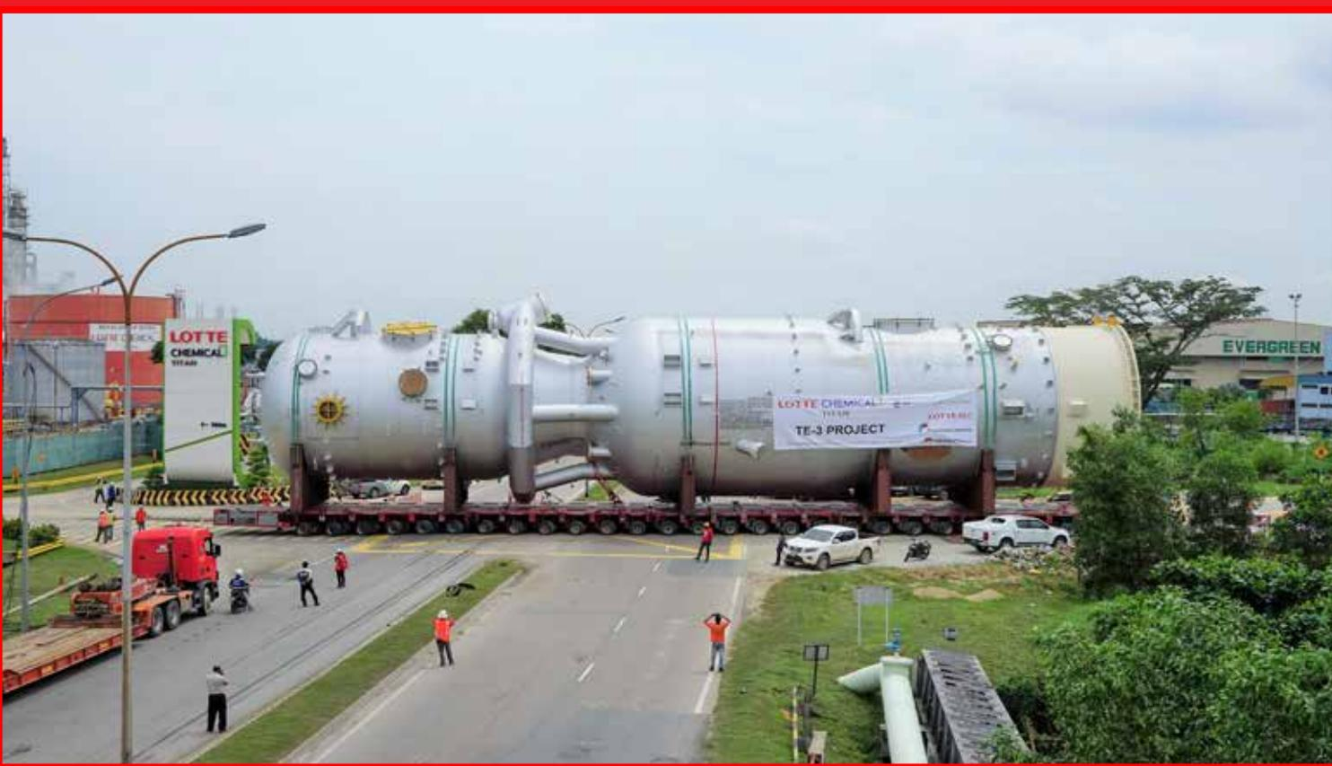
Another massive move by Megalift is the converter unit that weighed 709 tons, also from Pasir Gudang container wharf to Lotte's chemical site.
