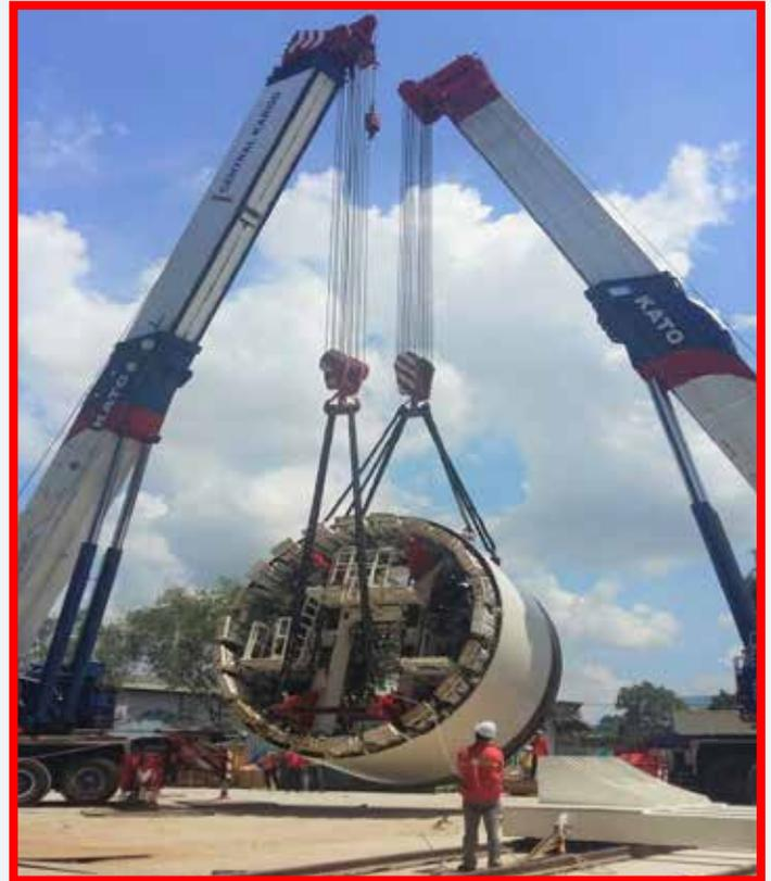
Cargo: Front Shield of Tunnel Boring Machine
