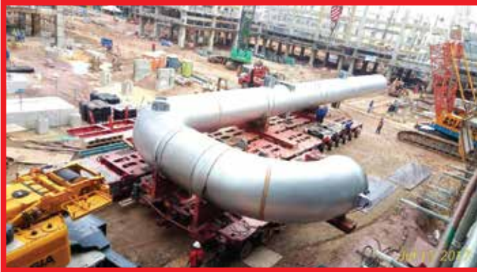
Cargo: Pipe Spool Dimension: L39.39 m x W12.15 m x H2.44 m Weight: 86 tons
