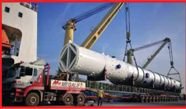
Cargo: CO2 Stripper Dimension: L75.30 m x W6.00 m x H6.40 m Weight: 233 tons
