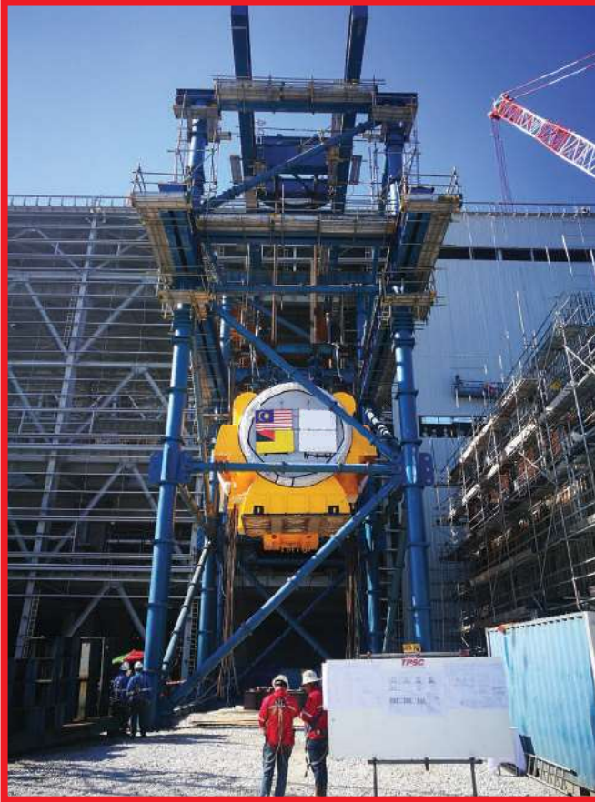
Cargo: Generator Stator Dimension: L10.95 m x W6.80 m x H5.47 m Weight: 462 ton Scope: Lifting, turning & positioning
