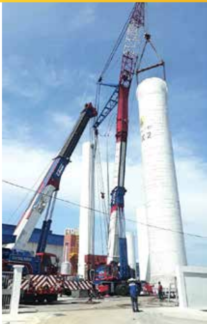
Lifting & Positioning to foundation
